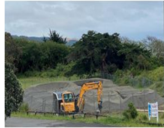
Photos of the Korora Park Pump Track under construction.
